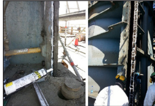
860 MPG applied to the door flanges and mill housing.
